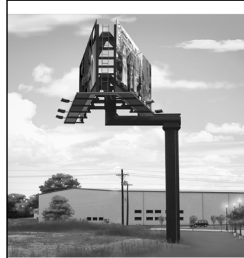
The offset column supporting this sign is subjected to the combined loadings of normal force, shear force, bending moment and torsion.
