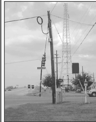
The long-term application of the cable loading on this pole has caused the pole to deform due to creep.
