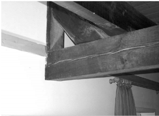
Typical shear failure of this wooden beam occurred at the support and through the approximate center of its cross section.
